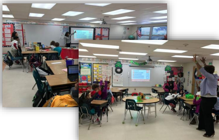
Coral Cove Elementary (District 2) – Ceiling projectors
